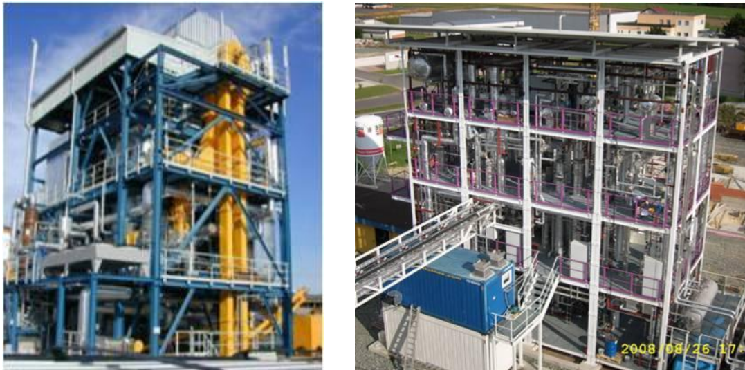
Figure 3: REPOTEC-CTU's 8MW th FICFB gasifier (left) 14, and 1MW bioSNG methanation unit (right), installed in Güssing, Austria 15
