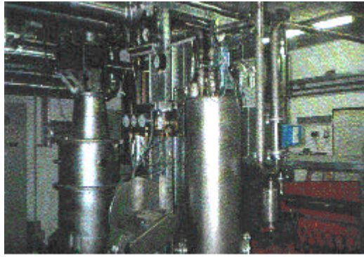
Wood gasifier for co-gen set
