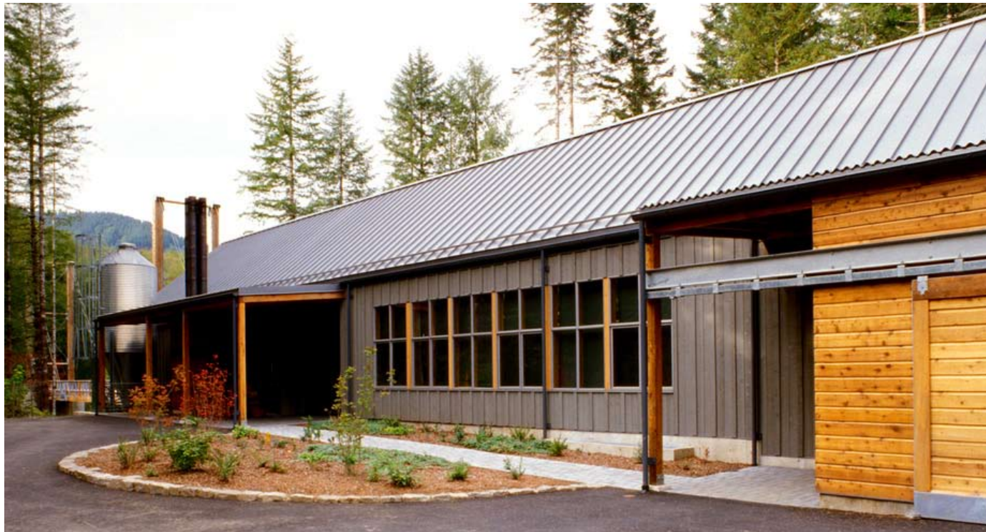
The storage silo for pellets is accessible, but unobtrusive towards the rear of the building. Photo: Oregon Dept. of Forestry.
