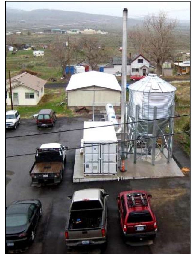
The entire system, including storage silo, occupies a total of four parking spaces. Photo: Harney District Hospital.
