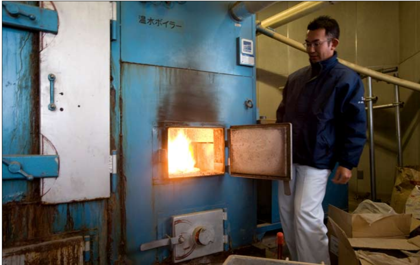
Consistent size, shape, and low moisture content ensure wood pellets burn efficiently in this wood pellet boiler. Photo: Dan Bihn
