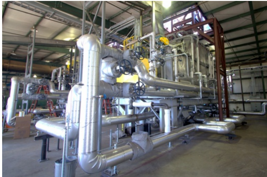
Figure 7.7 The NBE torrefaction Reactor
