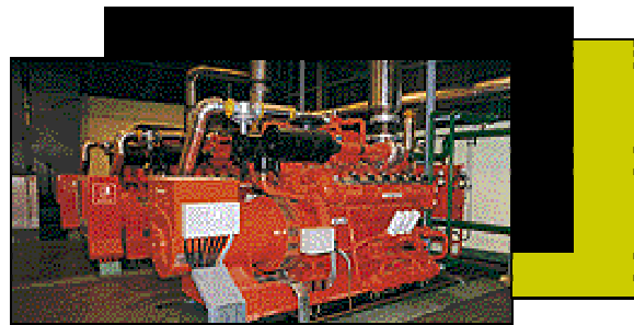
Guascor Gas Bio-gas Gensets
