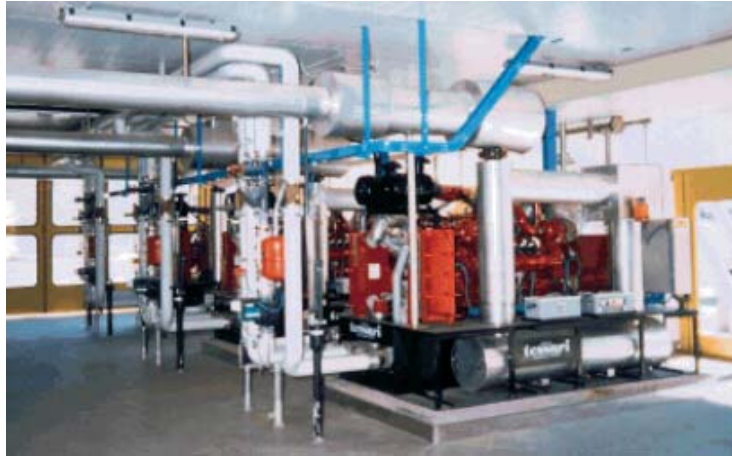
Tessari's cogeneration-sets with 8-cycle engine fuelled with biogas. Electric continuous total power 450 kW a power factor 0.8 and thermal power 780 kW.
