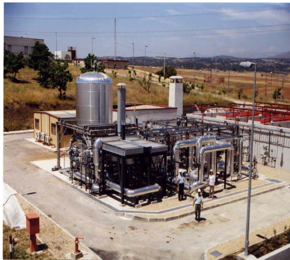
PEP Iberdrola station test at S. Augustin de Guadalix (Madrid, E)
