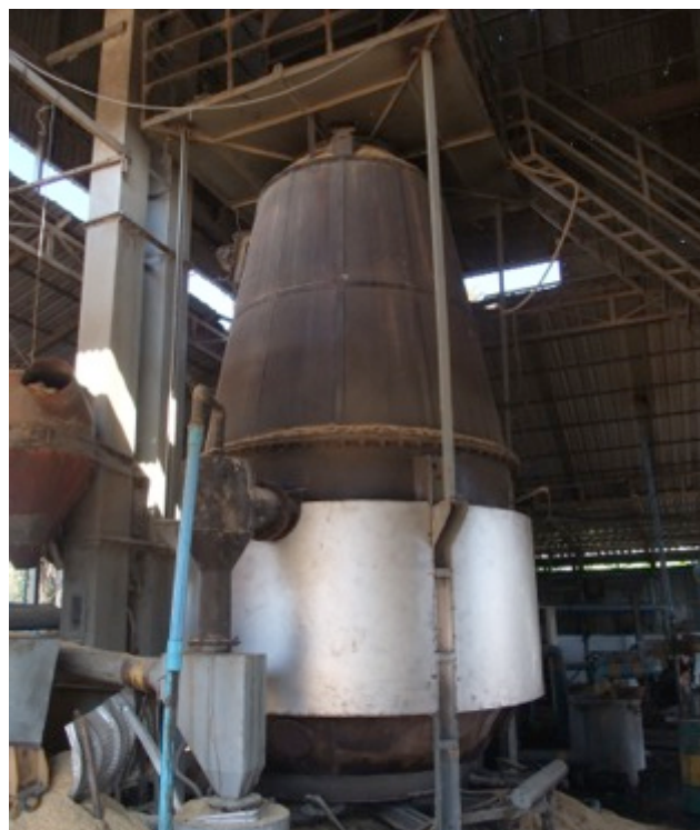
Figure 5: 600kW gasifier, local manufacturer at Yam Chan rice mill, Battambang province, Cambodia, 2014 - 12 – 20
