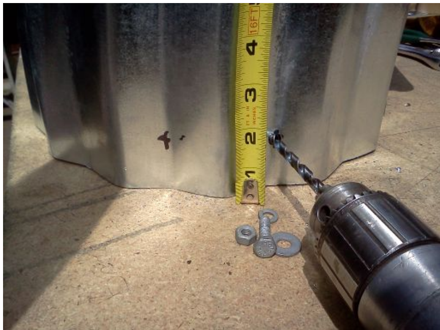
1/4in nuts and bolts 1-3/4in up
