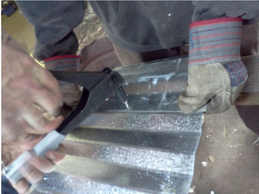
Drill & Rivet ends & center in turn
