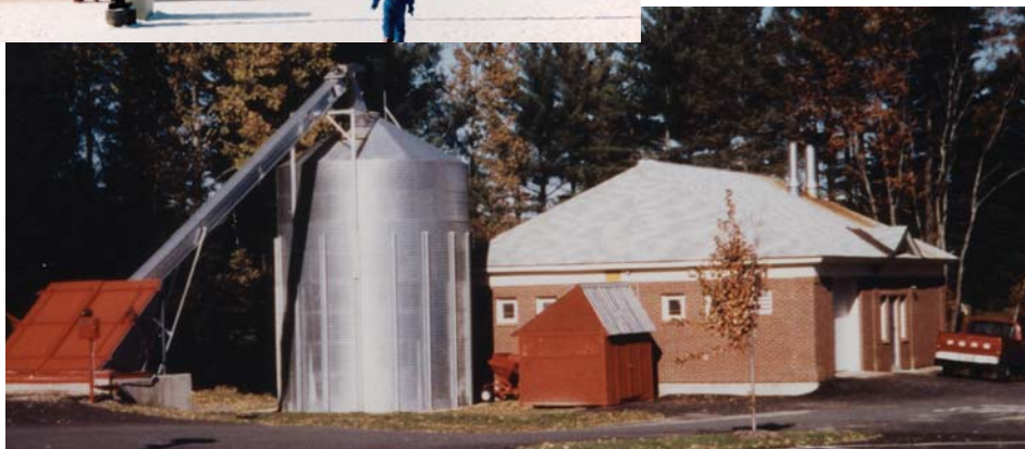
Lyndon Town School, Lyndon, Vermont System Size: 1.2 MMBH Manufacturer: Chiptec Wood Energy Systems This system uses an above-grade metal silo and separate boiler house (which includes garage space). Silo is loaded from a receiving bin (on far left) using an inclined auger.
