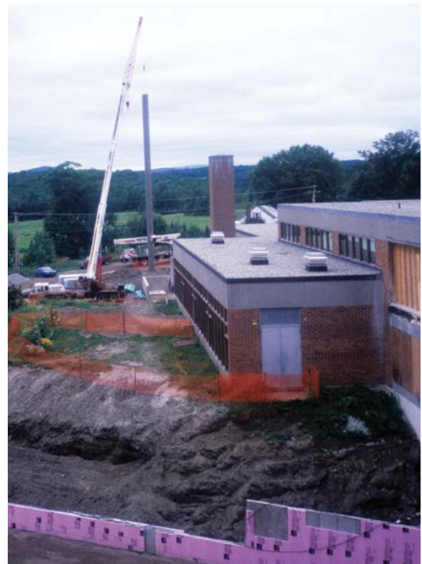
Union 32 Junior-High School, East Montpelier, Vermont. 4.5MMBH Manufacturer: Messersmith Manufacturing Installation of a tall stack.
