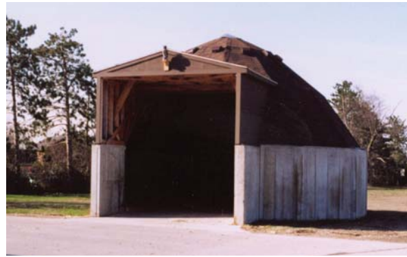
Camp Johnson, Essex, Vermont Facility Type: National Guard base System Size: 3 MMBH
