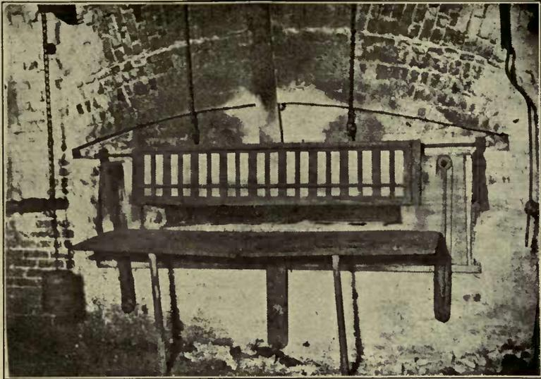
FIG. 140.—Producer Gas Heating Furnace for Heating Plates for Pressing into Shapes.
