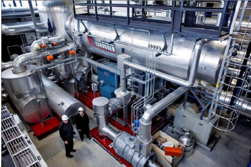
Figure 14. Turboden ORC plants are factory installed on the platforms, and during the assembly in the CHP plant they are connected together and to the boiler. The ORC-CHP plant in the picture is in Toholampi, Finland, and the power output is 1.3 MWe. Photo: Turboden.it
