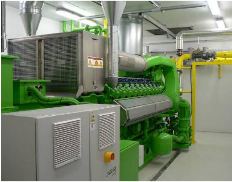
Figure 17. IC gas engine ( piston engines ). Example of a piston engine in a CHP unit, a 20-cylinder Jenbacher gas engine.
