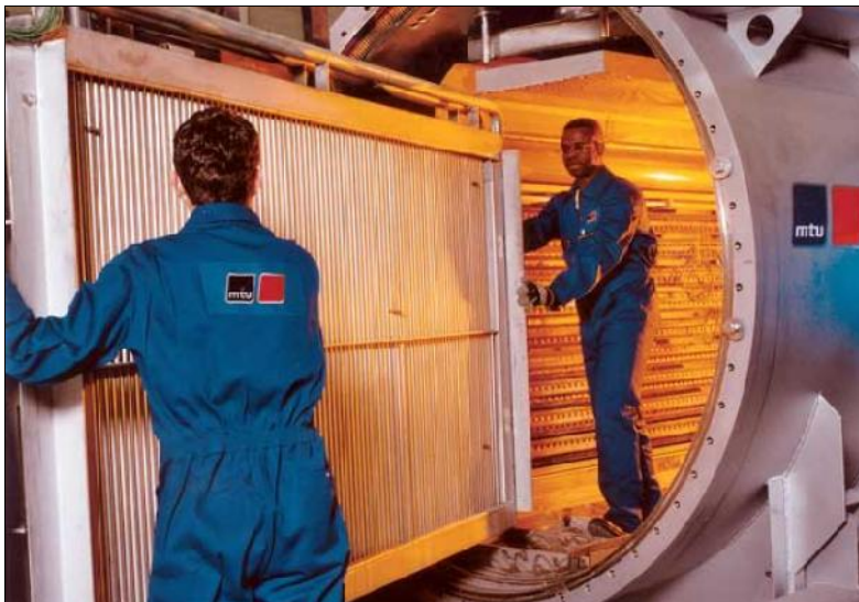
Figure 18. Installation of a fuel cell stack at a MTU CFC plant in Germany.
