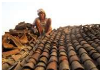
Picture 19 The broken pottery roof tiles
