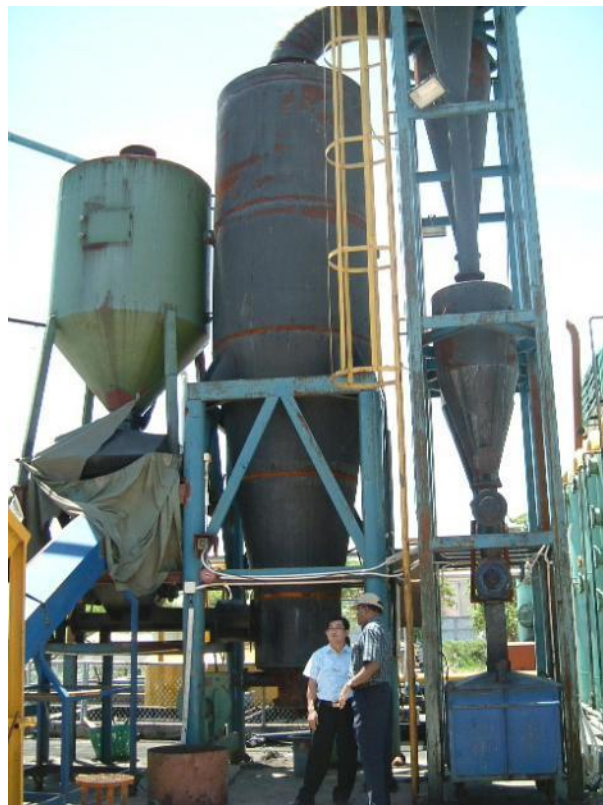
Waste plastic gasification plant at Samutsakorn
