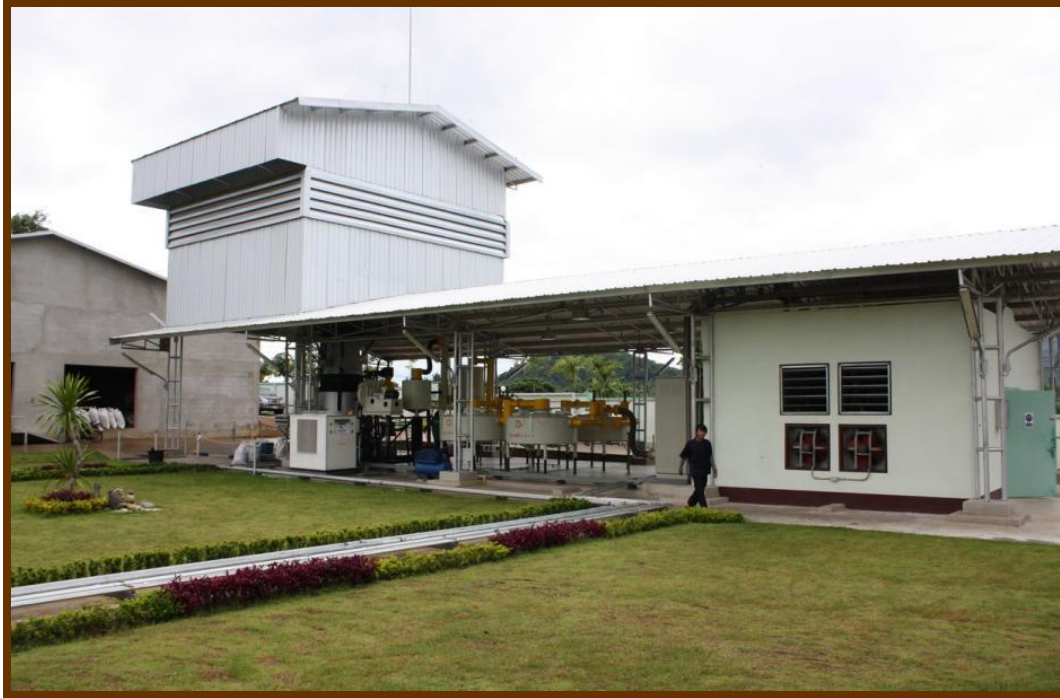
Supreme gasification power plant
