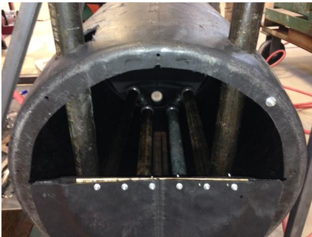
Figure 2-6 Steam Feed Heat Exchanger Interior
