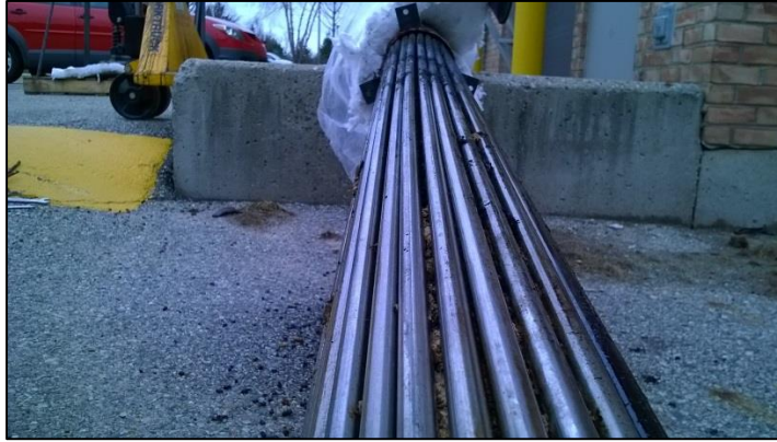
Figure 4-5 Pipes in Disassembled Gasifier
