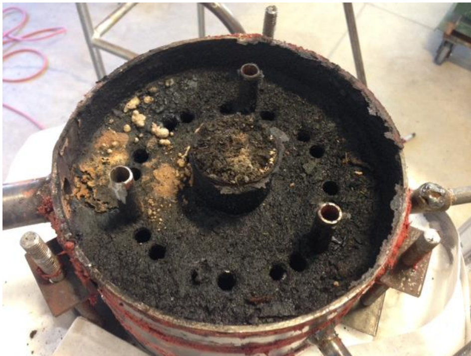
Figure 4-4 Synthesis Gas Manifold with Tar Deposits
