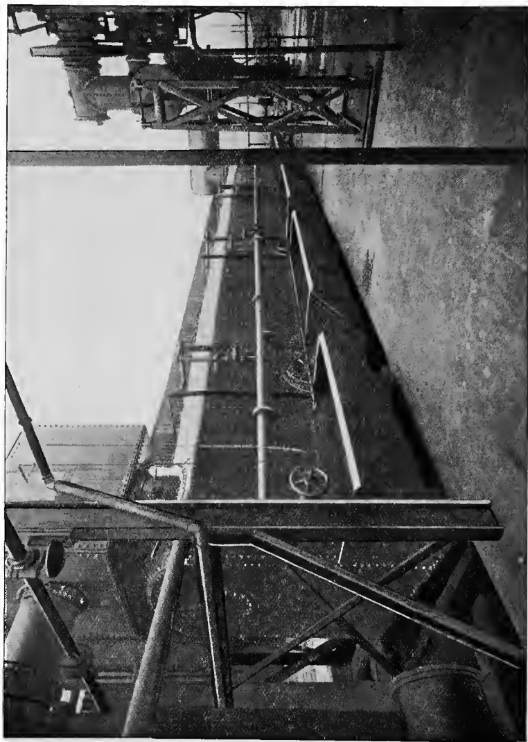
FIG. 98. Mechanical washer for 3000 B. H. P. gas plant.
