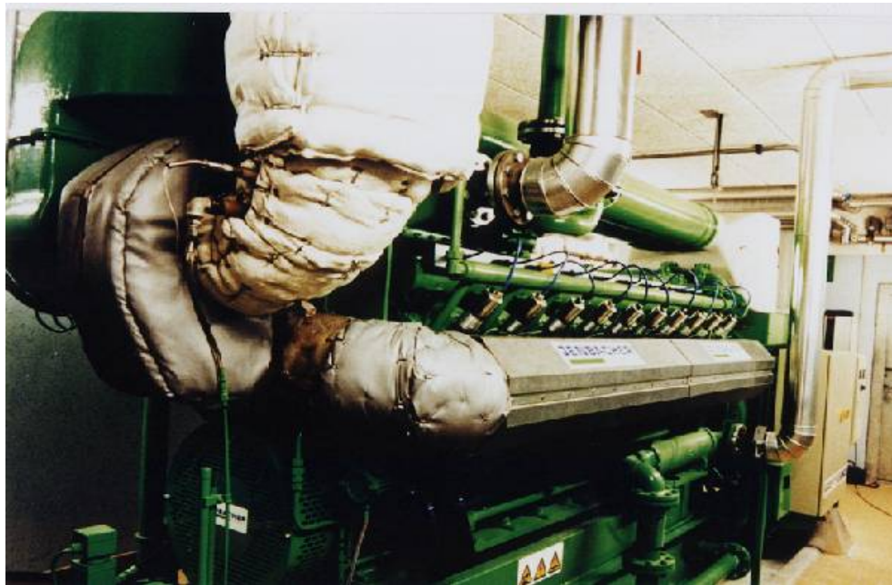
Figure 7.13. Jenbacher engine at the Harboøre plant (courtesy of GE's Jenbacher gas engine business) [19].
