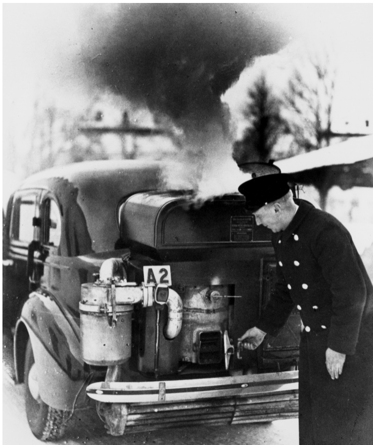
Figure 6.8. Private car wood gasifier. To operate the system, the driver periodically had to feed the gasifier with wood pieces. This particular car belonged to the Swedish King (Copyright Scapix Sweden).
