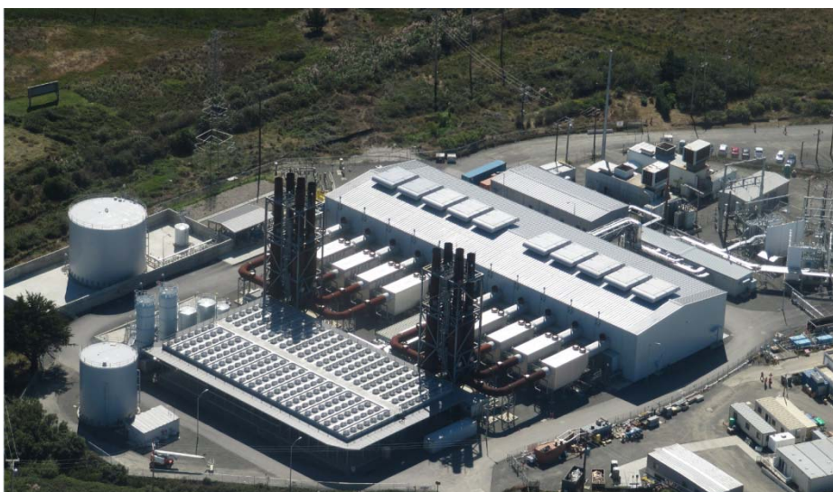
Figure 6.4. The Humboldt power plant in California consists of ten Wärtsilä dual-fuel gas engines with a total output of 162 MW. To meet the strict Californian emission requirements, SCRs are employed (courtesy of Wärtsilä) [7].
