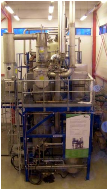
Figure 7.4. MEVA Innovation's 500 kW VIPP-VORTEX pilot plant at ETC in Piteå, Sweden.
