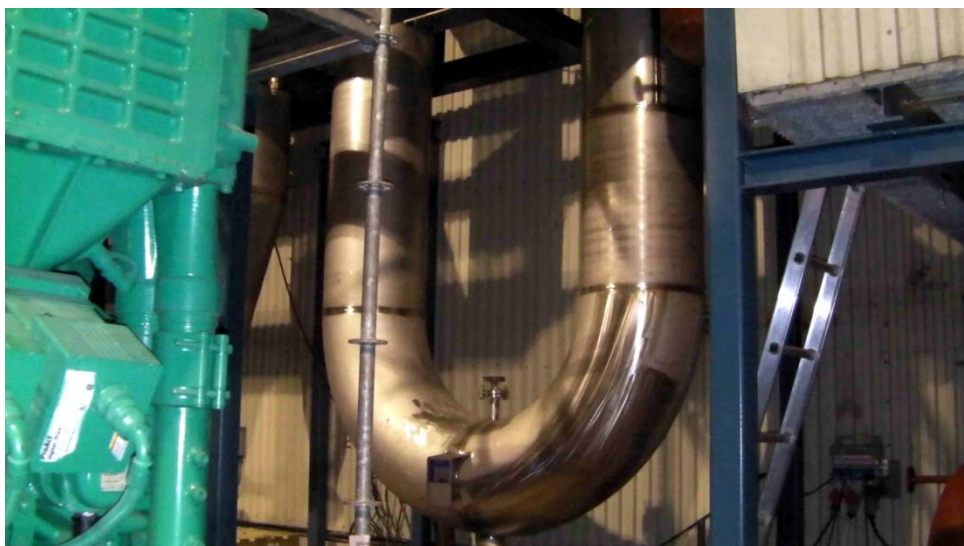
Figure 7.6. Unassembled parts of the Hortlax plant. The bio-oil scrubber is shown in the centre and the gas engine to the left in green.
