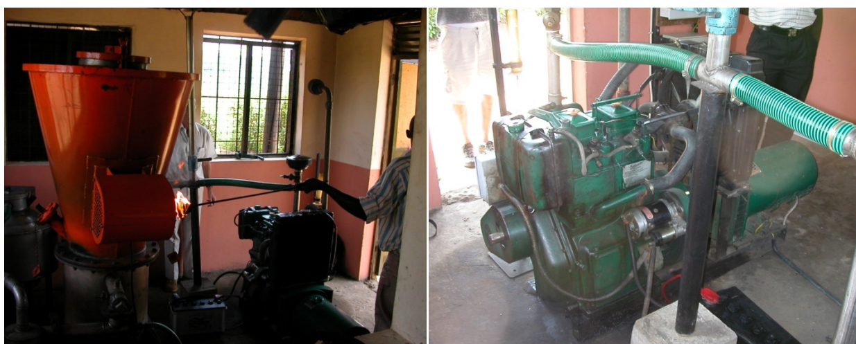
Figure 7.16. Gasifier (left) and gas engine (right) at Mukono, Uganda (photo courtesy of T. Buchholz).
