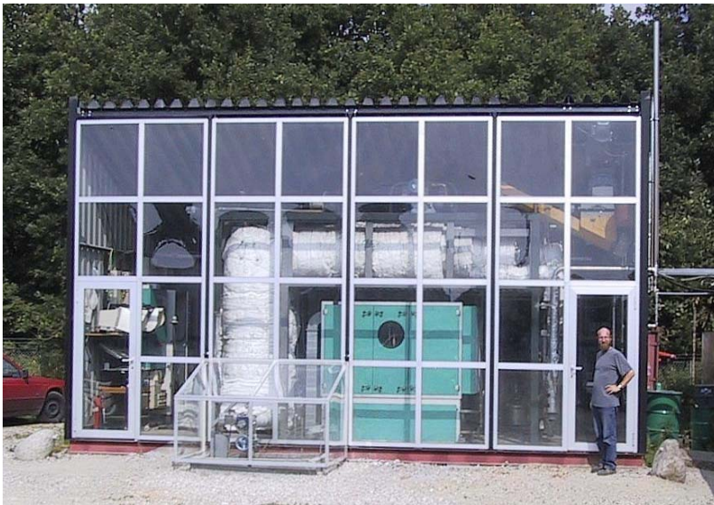
Figure 7.1. The Viking 80 kW th gasifier (today located at the Risø facility) (courtesy of the Biomass Gasification Group, DTU)
