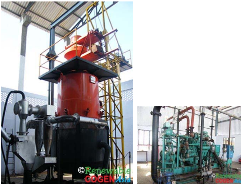
Figure 7.21. A 250 kW rice husk gasifier from Renewable Cogen Asia (photo courtesy of Renewable Cogen Asia).
