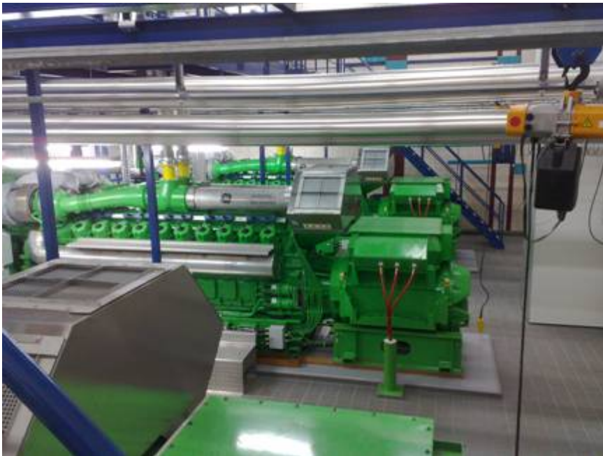
Figure 7.15. The three Jenbacher gas engines at the Skive plant (courtesy of GE's Jenbacher gas engine business) [19].
