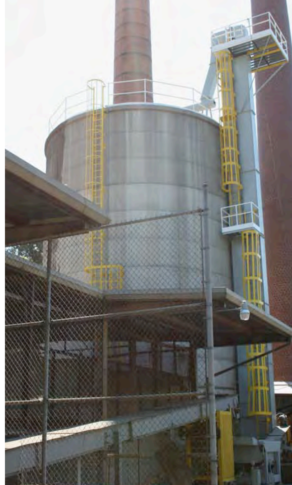
A direct combustion system fueled by wood waste with storage silo in foreground.
