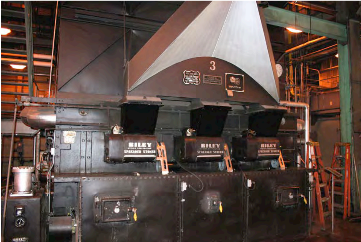
A spreader stoker coal boiler, a standard type of combustion system where co-firing will occur
