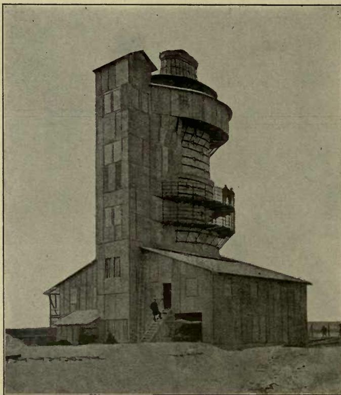
FIG. 174.—View of German Gas-fired Lime-Kiln.
