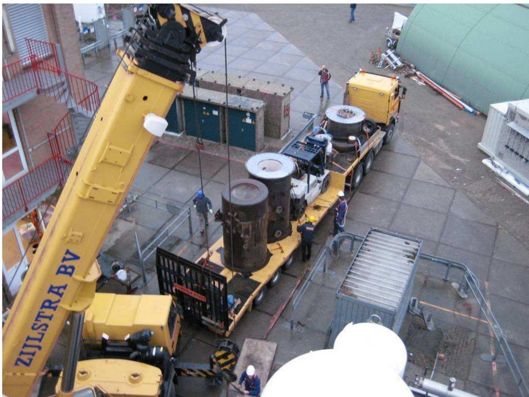
Figure 6-11: Arrival of the MILENA reactor segments at ECN.
