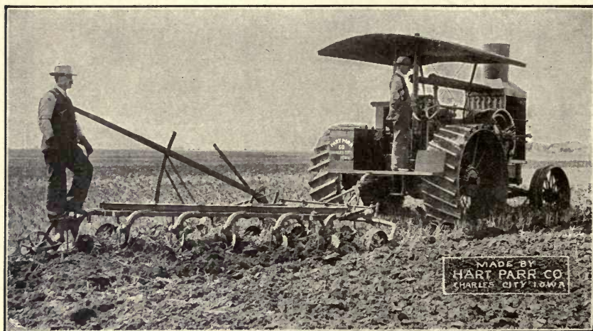
FIG. 112. — HART-PARR GASOLINE TRACTION ENGINE.
